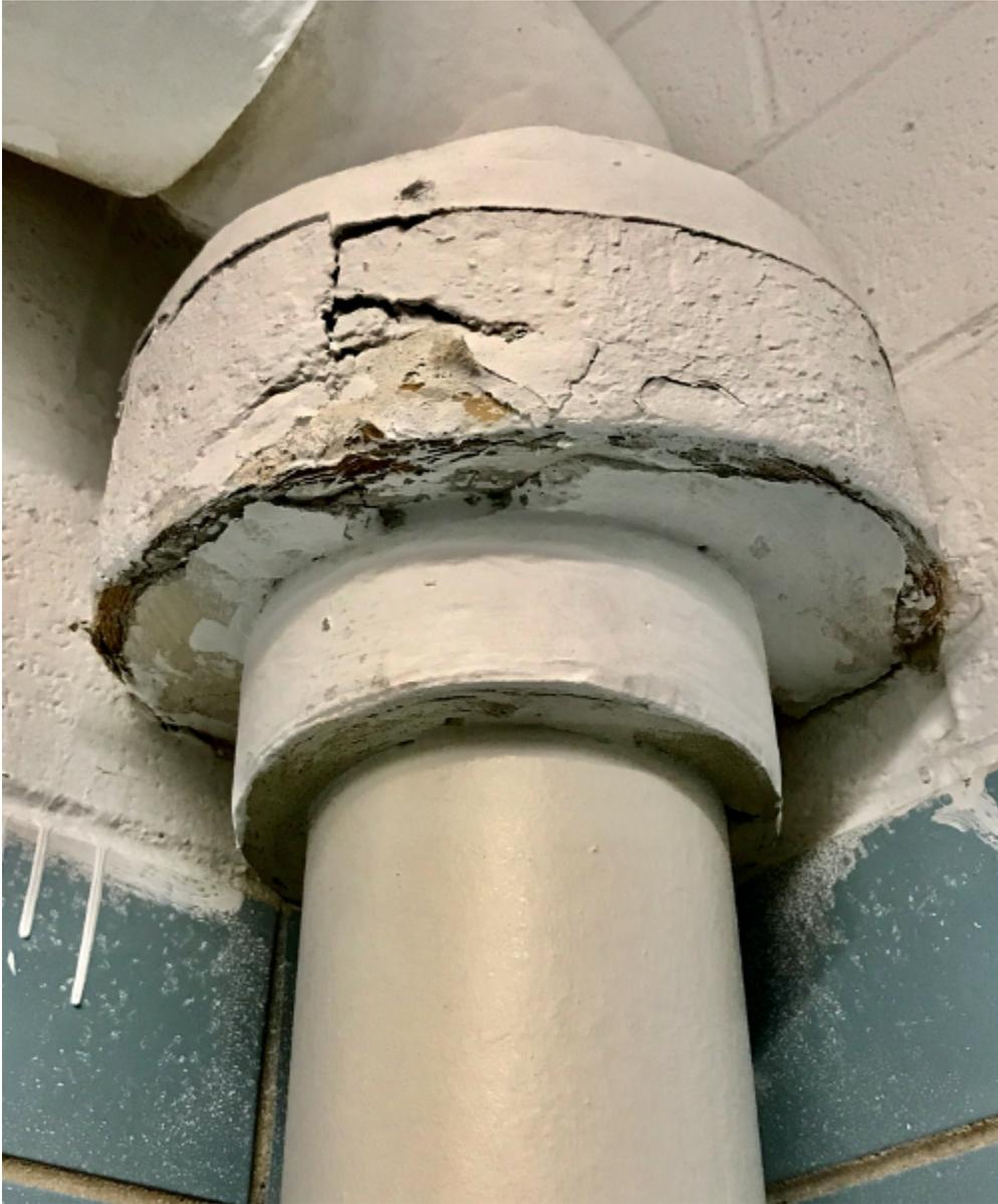
**Photo 19 – Bathroom (close-up of above) — Showing damage to asbestos insulation**
