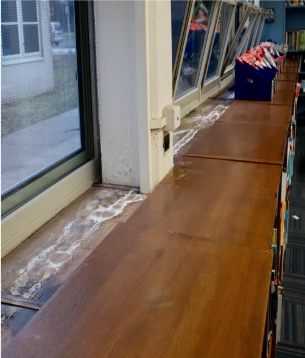
**Photo 13- ES Library** – Mold growth and damage to cabinets from ongoing and unrepaired steam leaks
