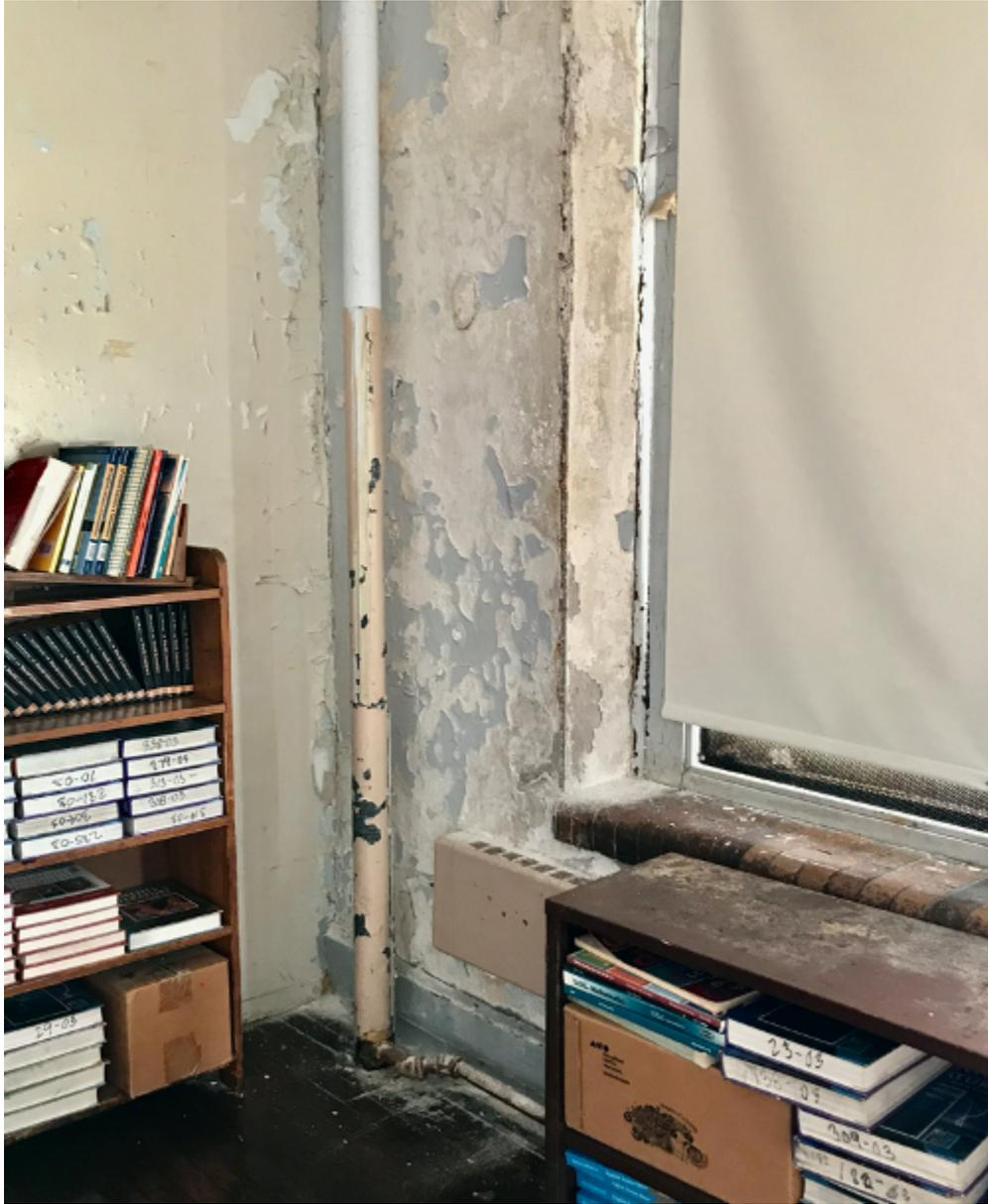
**Photo 2 -- ES Classroom — Extreme water damage resulting in severe deterioration of lead paint - flaking with dust and debris on materials**
