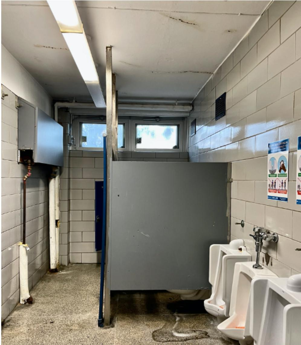
**Photo 16 – Boys Bathroom (ES) — Filthy conditions - leaking on floor and ceiling - deteriorated/damaged and missing insulation on piping presenting a burn hazard from very hot heating pipes**
