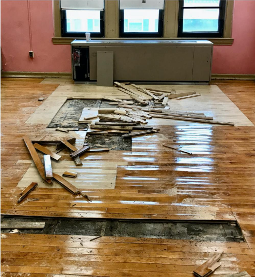
**Photo 9 – ES Classroom** — Repeat flooding from malfunctioning classroom unit ventilator resulting in extensive damage and mold growth to newly installed flooring — the original flooring was replaced for the same reason just a few weeks earlier. An example of what happens if the “root causes” are not addressed and also issues related to inadequate governance, oversight, and management
