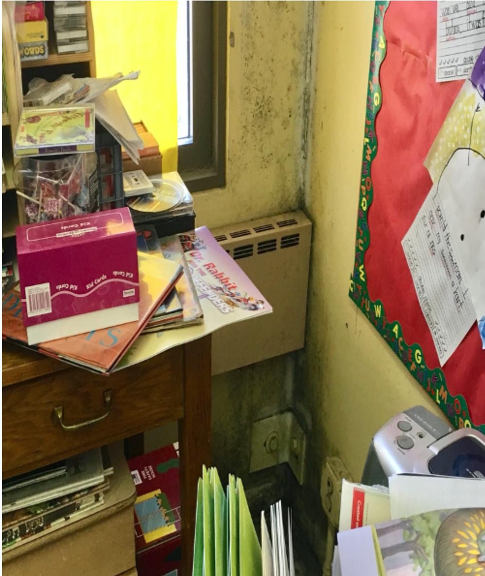
**Photo 7 – Mold Growth on Wall of Occupied ES Classroom — According to Classroom Teacher This Condition Had Been Present for Several Months — Associated with HVAC System Problems**
